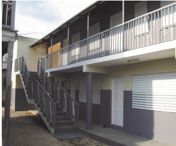
New classrooms in final preparation at East Street
